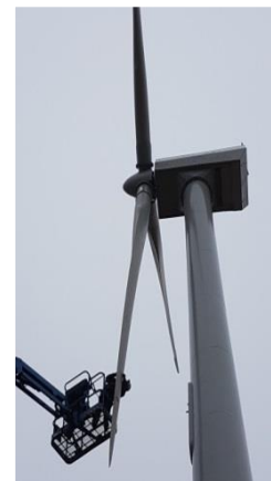
Blade tip repairs
