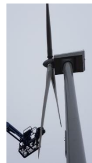
Blade tip repairs
