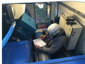
Scheduled servicing to manufacturer's protocols
